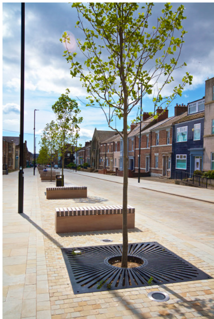
Photo 4.1: Howard Street, North Shields
